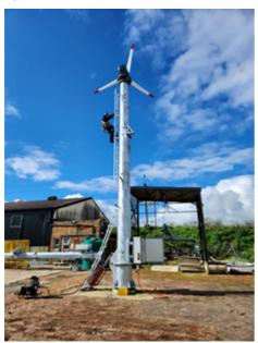
The 30kW model is their flagship frost fan; its reach extends to 9 hectares and runs at 800 revolutions per minute, which means that noise can be a factor.
