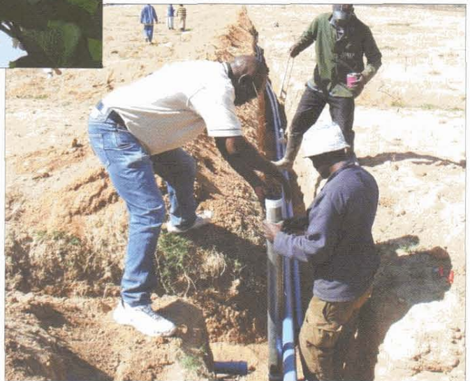
Green Mbhalati with workers installing new micro-jet irrigation lines.
